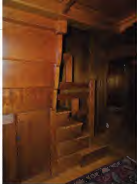
Work in progress. The second-floor stairs in Charles Greene's home were added in 1906. The house was in constant flux, growing with Charles' family.
